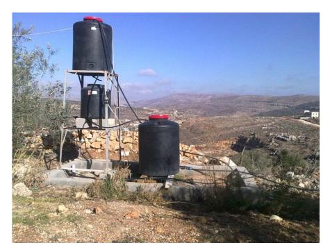
Photo 2-2 Onsite grey water treatment plant, Duara AlQare'- Ramallh, 2011
