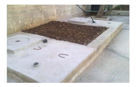
Photo 2-5 Onsite grey water treatment plant after finishing works, Jifna-Ramallh, 2010
